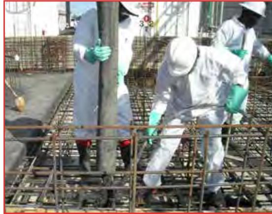
**TUFCEM™ Silicate Concrete** is an acid-resistant substitute for Portland cement concrete. This active pharmaceutical ingredient plant, which uses strong sulfuric and acetic acids, constructed secondary containment dikes using TUFCEM™ Silicate Concrete that was mixed on site in a continuous volumetric mix truck.
