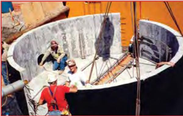
**Urethane-asphalt TUFCEM™ II Membrane** was used to coat the exterior surface of this sulfur pit made of **TUFCEM™ Silicate Concrete**. The sulfur pit was precast in two pieces then joined in the field.
