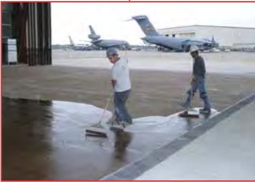
Aircraft maintenance facilities utilize aggressive chemistries for parts and engine cleaning and paint stripping. Properly selected **PENNCOAT™ Lining** or **PENNTROWEL™ SB Flooring** provides effective concrete protection in these facilities.
