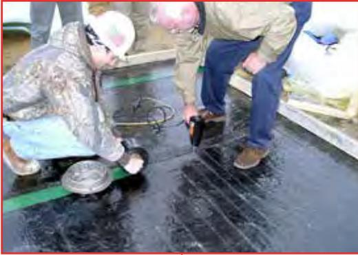
When installation time is limited, consider a pre-cured, adhesively bonded sheet membrane like **PENNCOAT™ 600 Membrane**. Seams are sealed with heat and chemical-resistant tape.
