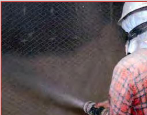
In predominantly hot and dry stacks, plural component **TUFCEM™ Silicate Gunite** lining is an economical choice. For best performance, the substrate and anchoring system are first lined with a chemical-resistant membrane, such as **PACMASTIC™ 325**, prior to installation of the gunite.
