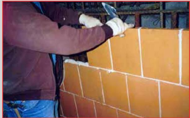
Vinyl ester mortars have historically been used in tile-lined, pulp bleach plant equipment. Our family of **vinyl ester PENNCHEM™ Mortars** provides customized performance to address variations in pH and temperature for optimal mortar longevity.
