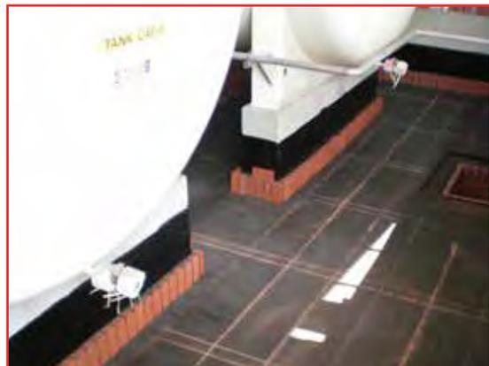
This lead-acid battery manufacturer protects its strong acid storage and mixing containment areas with **acid brick** and **FURALAC™ Green Panel Mortar** over **asphaltic PENNCOAT™ 101 Membrane**.
