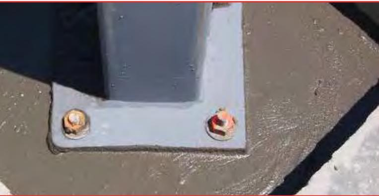
■ Column base plates need solid support for efficient load transfer. High-strength **TUFCEM™ Grout** is a great choice for pours up to one foot deep.
