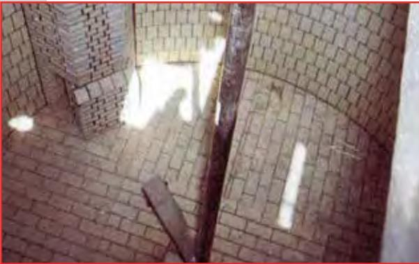
Historically, **brick linings** are utilized in the most demanding environments, and provide reliable service with minimal maintenance.
