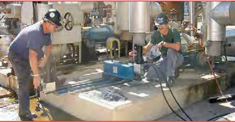
■ **TUFCEM™ Silicate Concrete** offers unmatched resistance to strong nitric, sulfuric, phosphoric, and hydrochloric acids. Construction tools and techniques are similar to those used for conventional Portland cement concrete.
