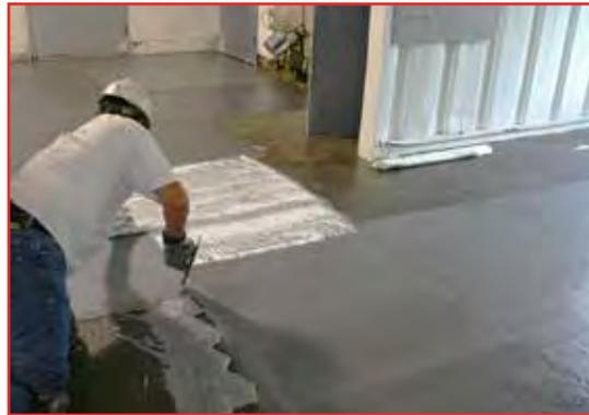
Compared with trowellable PENNTROWEL™ Surfacers Systems, **PENNTROWEL™ SB Systems** are applied using less labor-intensive slurry-broadcast installation techniques. These methods yield a non-slip, durable broadcast floor finish.
