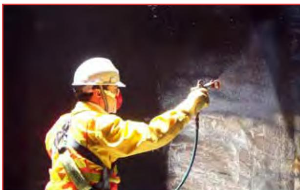
The elastomeric nature of **TUFCEM™ II** and **PENNCHEM™ 97 Membranes** allow them to accommodate some movement in the substrates over which they are applied. Both are useful secondary containment linings.
